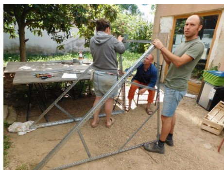
Montage structure acier
