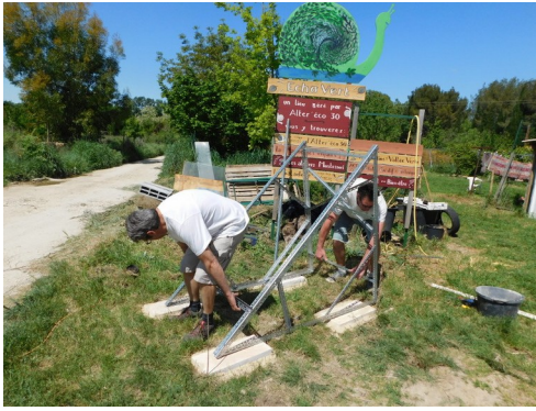
Pose structure acier
